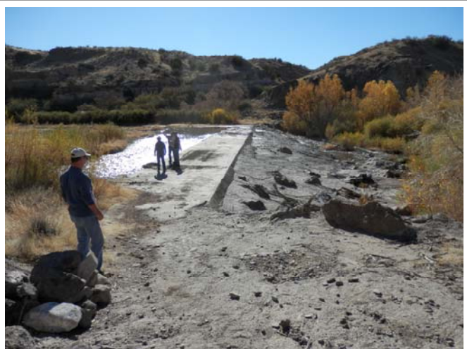
Weir type diversion structure located near Virden, NM
