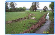
Ditch (Acequia) A structure used to convey water to a tract of land for irrigation purposes.
