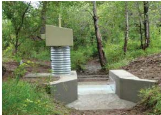
This Acequia Madre de Los Vigiles Flume at Rio Gallinas (left) and the lower staff gage (right) are two types of water flow measuring devices used to measure the flow of the water that goes through them or over them. The public, as well as OSE/ISC staff, will soon be able to easily access a growing set of real-time water flow measurement data collected in various river basins. The information will be available on the Office of the State Engineer in late Spring of 2011.
