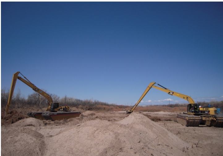
Amphibious excavators working in the river channel
