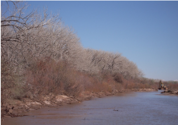
Before construction - March 2009 Bankline mostly Russian olive and Saltcedar
