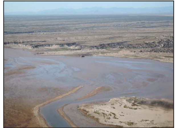
Aerial view of Pilot Channel in April 2003.
