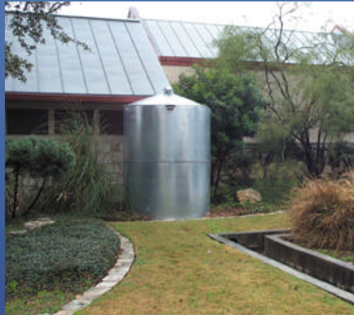
Rainwater harvesting storage tanks, such as this large galvanized steel cistern, should be located as close as possible to both the supply and the landscape where the water will be used.
