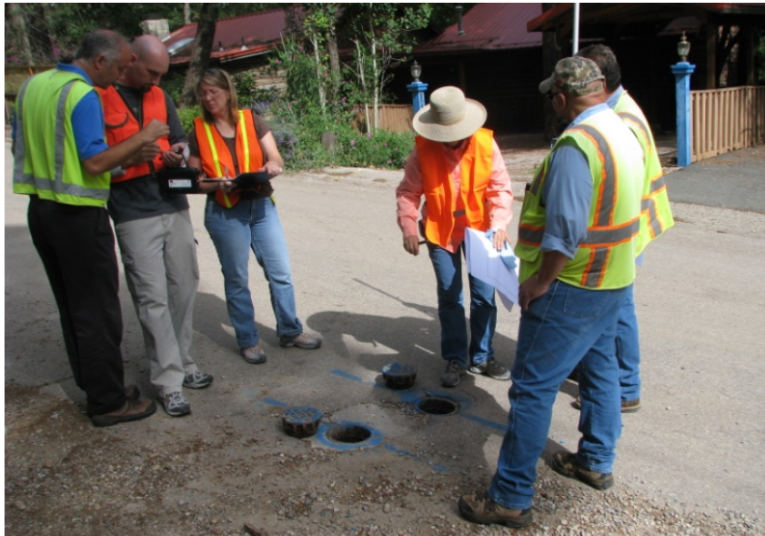
Figure 8: Ruidoso staff, OSE coordinator and consultants implementing the leak detection program.
