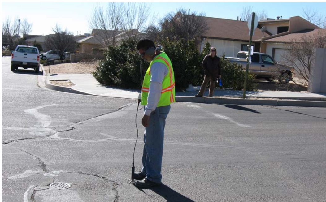
Figure 11: Rio Rancho personnel using ground microphone to listen for leak.
