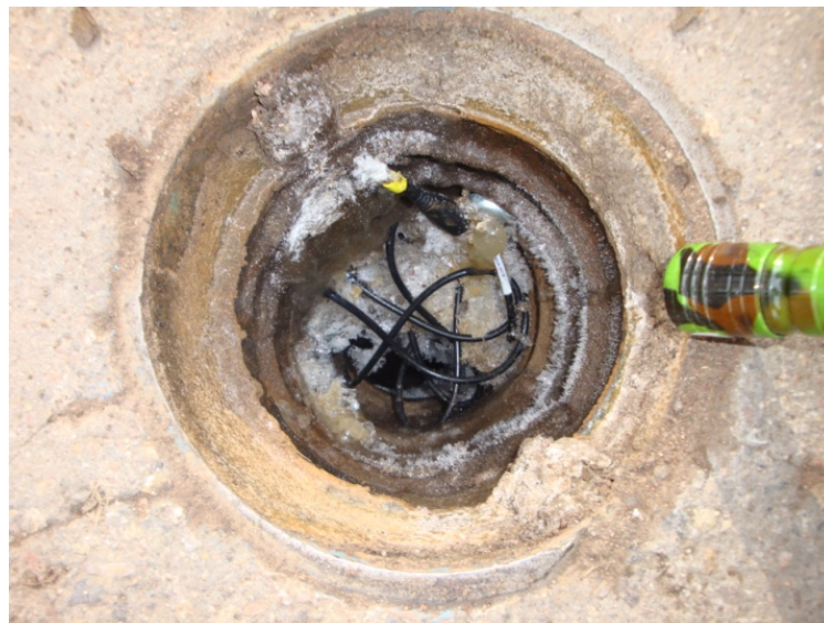
Figure 13: Ice filled valve box in Las Vegas, NM
