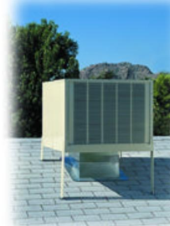
Virtually all models of evaporative coolers now available recirculate the water that drips from the pads, resulting in an efficient use of water. (Older, less water-efficient evaporative coolers might not have a pan to catch and recirculate water. These coolers should be replaced with recirculating coolers.)
