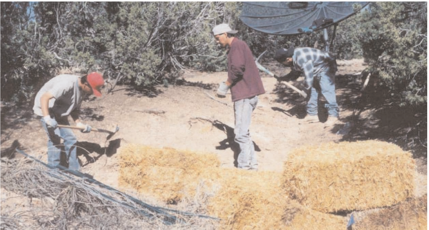
Figure 1-4: Workers install a straw bale swale.
