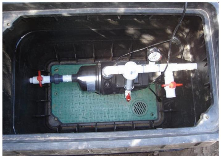
Figure 11-2: A good design narrative and an "as-built" manual will give an overview of the system and its components. Top: this purple valve box cover indicates the water in this system is nonpotable. Middle: a rainwater prefilter. Bottom: a pumphouse with drain pressure gauge and manifold.
