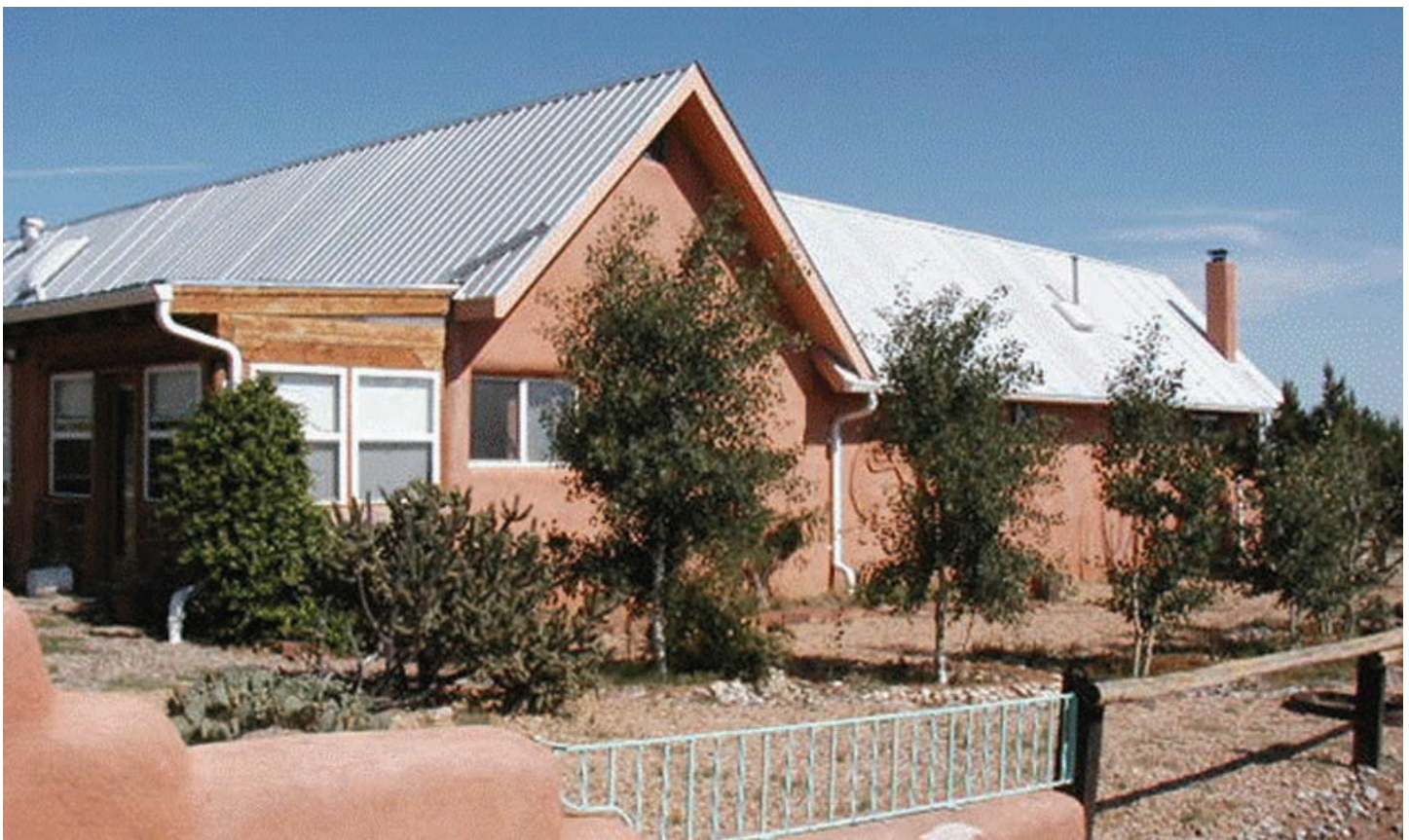
Figure 7-1: A pitched metal roof is the most efficient catchment surface for rainwater harvesting.
