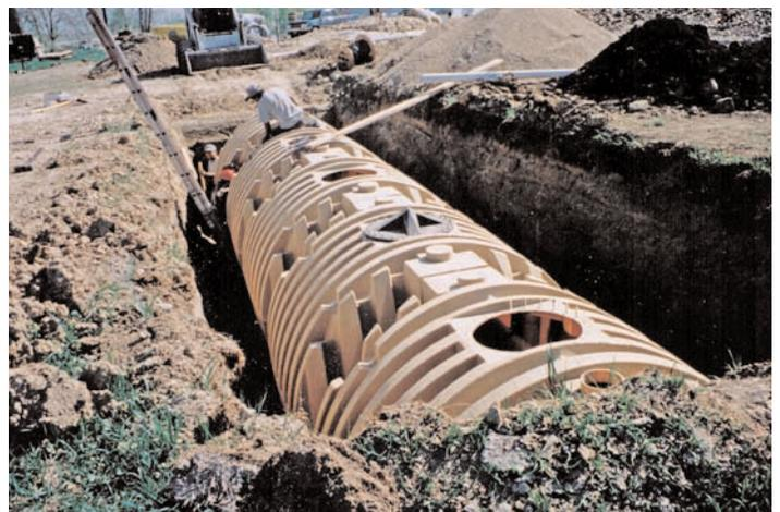
Figur 9-2: An underground cistern being installed.
