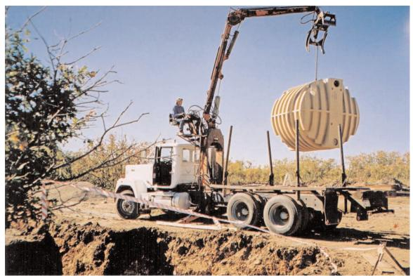
Figure 9-13: Large tanks must be delivered onsite via truck and lowered into place with a crane. The thick walls of this tank enable it to sit completely empty in the ground.
