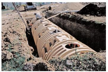
Figur 9-2: An underground cistern being installed.
