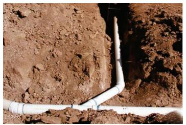
Figure 8-8: Conveyance pipes being installed, which will carry water to a cistern.
