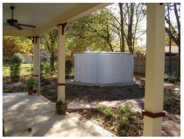
Figure A-2: A water storage tank is the heart of a roof-reliant landscaping system. Shown here is a 10,000 gallon aboveground corrugated metal tank.
