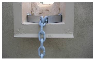
Figure 8-7: A rain chain is a simple but effective way to direct water downward from a canale.
