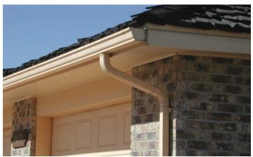
Figure 8-3: Photo of a downspout. Downspouts funnel water from gutters along a vertical drop.
