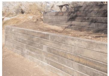
Figure 1-3: Retaining walls are an effective way to create terraces to control erosion and create spaces for plants.
