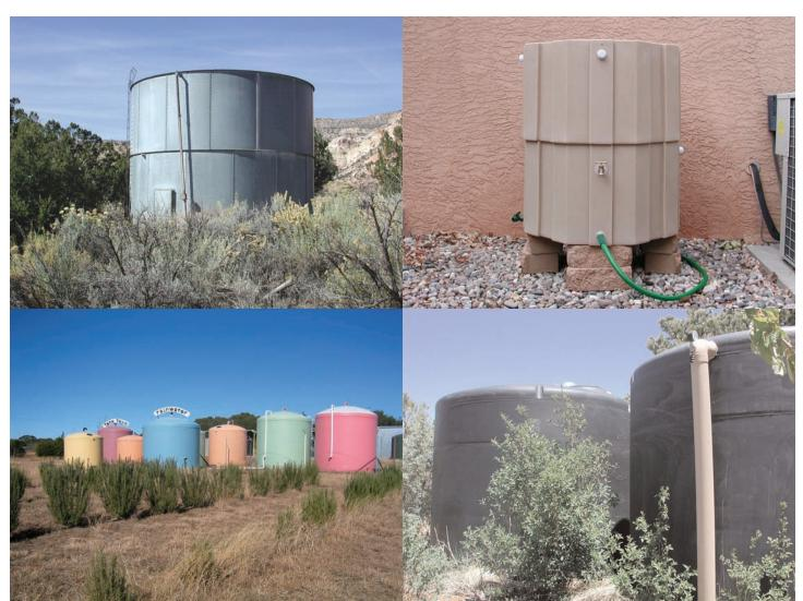
Figure 8-13: An assortment of water cisterns, clockwise from top left: a metal tank, two 54-gallon rainbarrels stacked on each other, two partially buried tanks, and an assortment of colorfully painted tanks.
