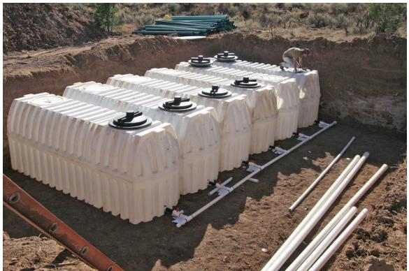
Figure 9-12: Tanks can be connected together to create larger storage capacity. These tanks will be connected in parallel, so that an individual tank can be shut off for maintenance or repair without disabling the entire system.
