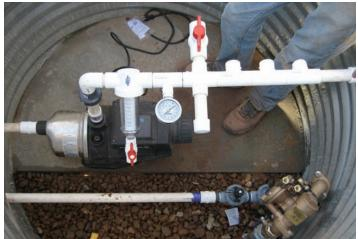
Figure 10-2. Sample inline pumphouse with spin filter manifold
