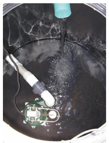
Figure 10-1: A sump pump must be submerged in water in order to work.
