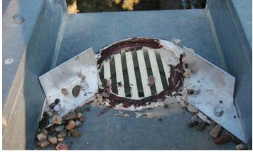
Figure 8-6: Partial dams installed on both sides of a drain directs the flow of rainwater.
