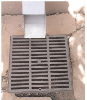
Figure 11-1: Leaf and debris screens and other filters need to be cleaned regularly.
