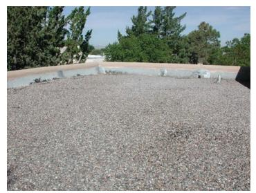
Figure 7-2: Although not the most efficient surfaces for harvesting rainwater, flat roofs can serve well as catchment areas for roof-reliant landscaping systems.
