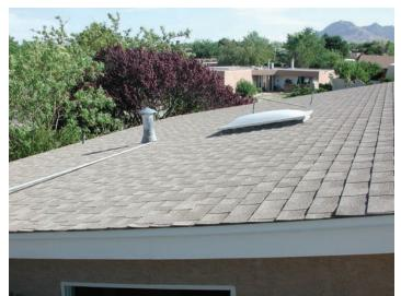
Figure 7-3: Asphalt shingle roofs, which are popular because they are relatively inexpensive, can be efficient for water harvesting.
