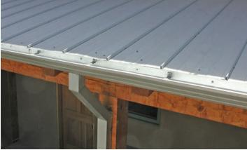
Figure 8-1: Gutters collect water from a pitched metal roof.
