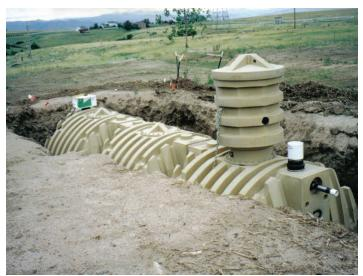
Figure 9-7: Once this underground cistern is installed and the hole is backfilled with dirt, only the serviceway will be visible.
