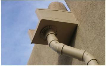
Figure 8-5: A toilet flange can connect a canale to a downspout.
