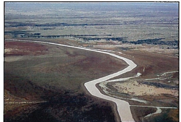
Aerial View of Completed Pilot Channel in February 2004
