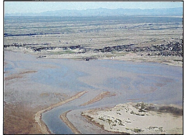
Aerial view of Pilot Channel in April 2003
