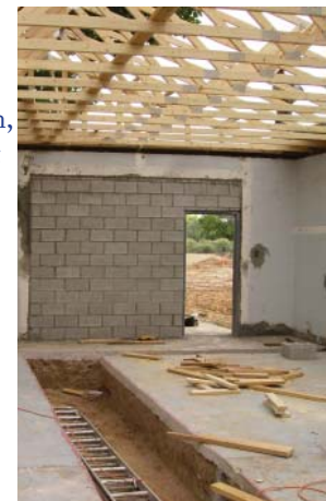
Main indoor drainage channel under construction at the refugium
